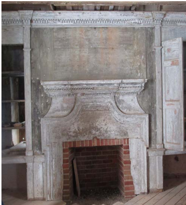
Original woodwork in the glebe house
