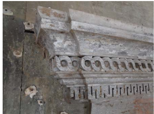
Detail of original woodwork
